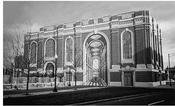
Figure 3. P S E & G Substation. New Brunswick NJ1982. Haas. http://www.richardhaas.com/
