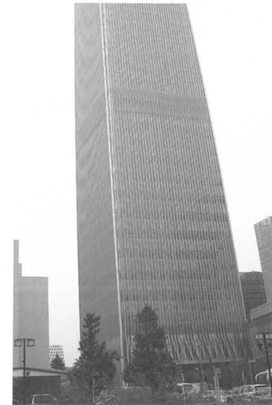
Figure 4.18. China World Trade Centre Tower 3.
