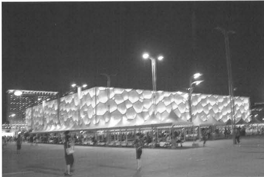
Figure 4.31. The Water Cube.
